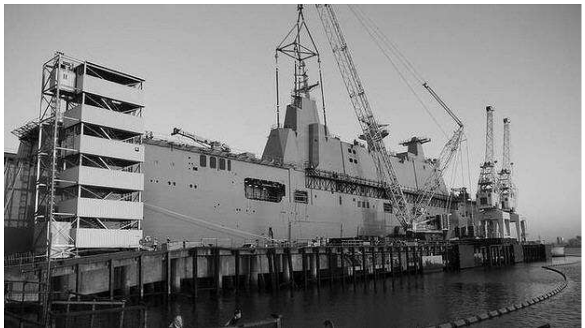
RIGHT Superstructure in place.
