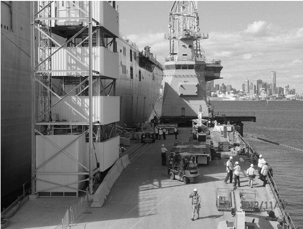
LEFT Superstructure block ready to be lifted to the deck.
